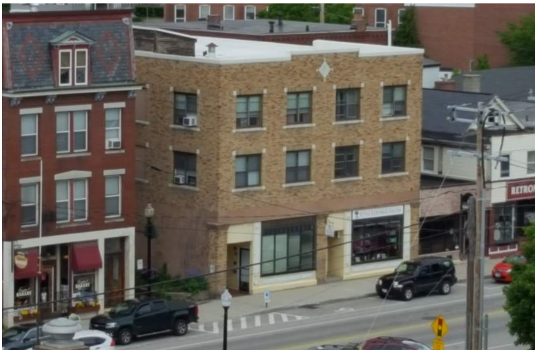
FIGURE 2: BENNETT BLOCK - FRONT ELEVATION, VIEW FROM WASHINGTON STREET
