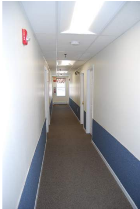
FIGURE 8: TYPICAL CORRIDOR - CARPET TO BE REPLACED WITH LVT.
