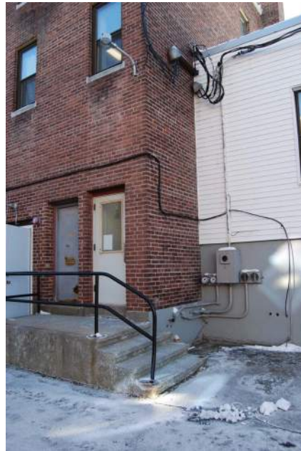
FIGURE 15: METERS AND SERVICE NEEDS TO BE MOVED OFF OF ADJACENT PROPERTY.
