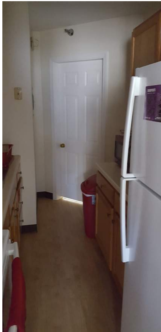
FIGURE 13: TYPICAL VIEW FROM INSIDE APARTMENT OF SPRINKLER COVERAGE ENDING AT ENTRY DOOR.
