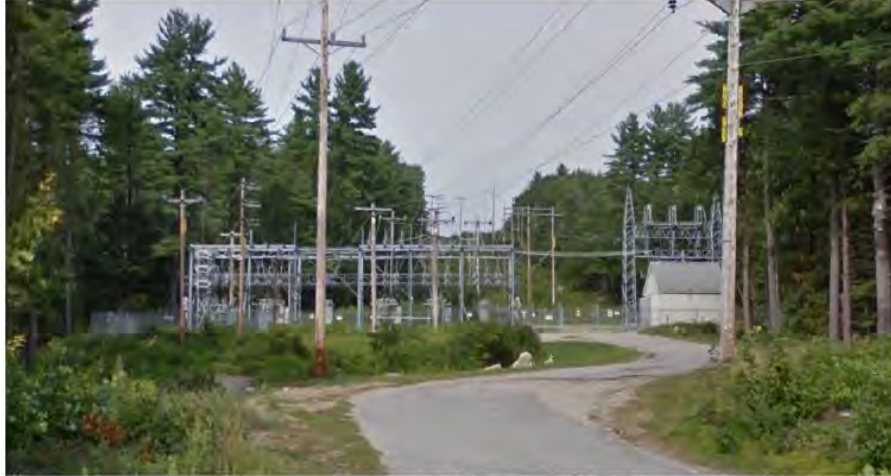
Figure 1. South Milford Substation viewed from Hammond Road, Milford.
