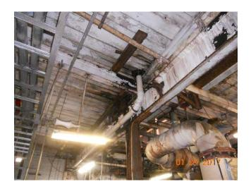
**Fan Room:** A door access through a masonry wall was found to be defective. Steel framed support channels were added to reinforce the opening as recommended in the original report. The photo below documents this installation.
