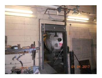
**Support of Coal Bunker Wall Opening:** A door opening which was cut through a thick concrete wall of the old coal bunker was found not to have proper support. The photo below shows two heavy gage pipe columns which were added to support the wall header above the door.
