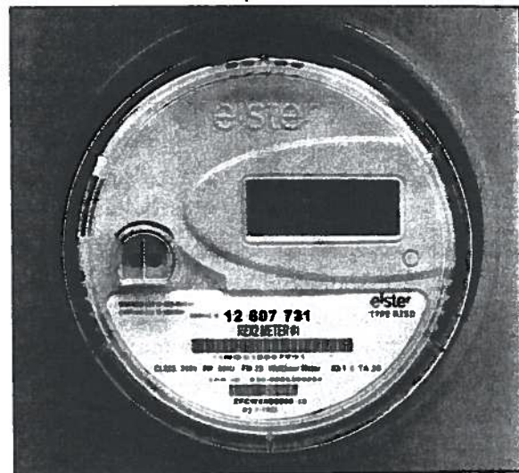
AMI meters look similar to the older electromechanical meters in use across Co-op service territory. Instead of gears and dials, AMI meters use a digital display to measure electric usage. A small transmitter in each meter sends usage data several times a day.
