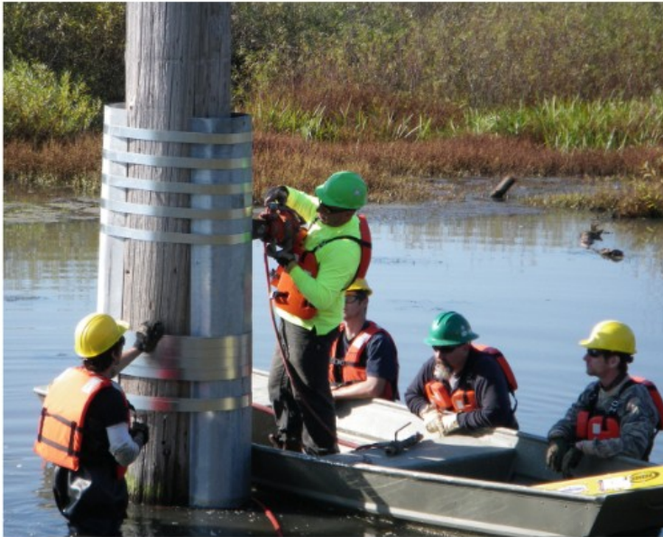
Poles in difficult locations such as hillsides, backyards or other difficult-to-access areas can be trussed to avoid costly, time-consuming replacements.
