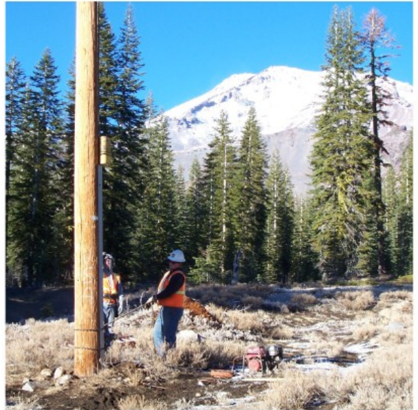
Poles in difficult locations such as hillsides, backyards or other difficult-to-access areas can be trussed to avoid costly, time-consuming replacements.
