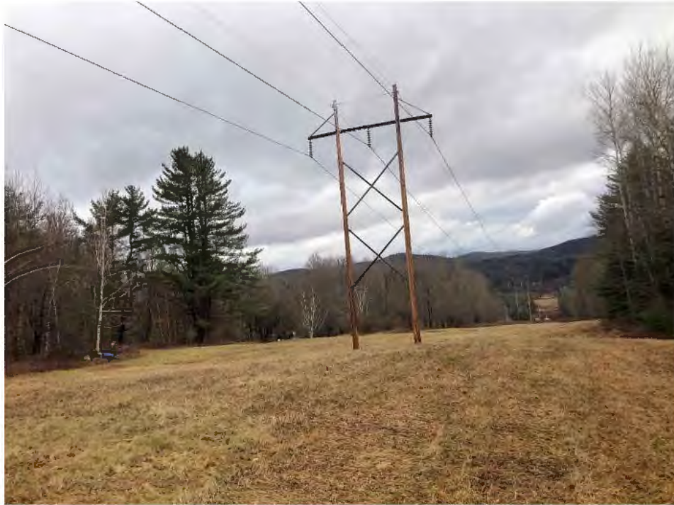
Photograph No. 98: Looking northeasterly at proposed access and work pad location for Structure 392.
