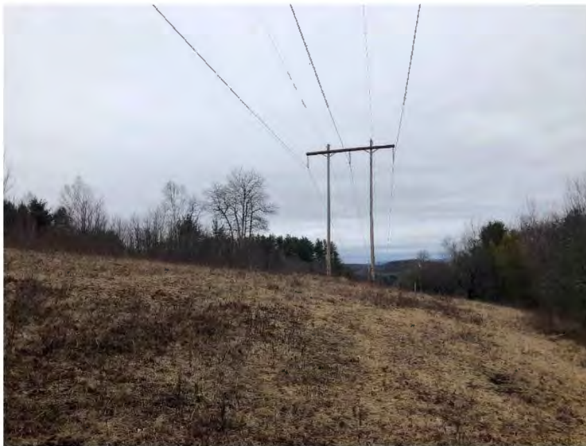
Photograph No. 95: Looking northeasterly at proposed access toward Structure 389.
