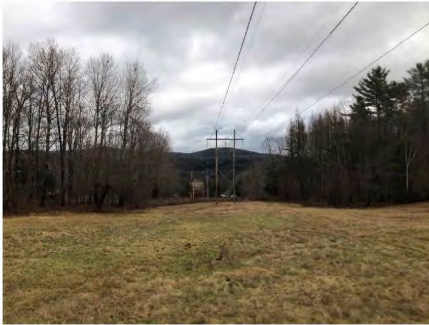
Photograph No. 99: Looking northeasterly at proposed access toward Structure 393.
