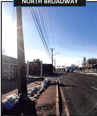
POLES 126, 125 East, 124 – behind backside sidewalk 126 – Double pole 125 East – Frontage issue redevelopment 124 – Double pole, new pole snapped POLE 123 – no clear space, visibility issue, traffic and safety hazard POLE 125 ON WEST SIDE: Service pole for Sal's and Depot Building
