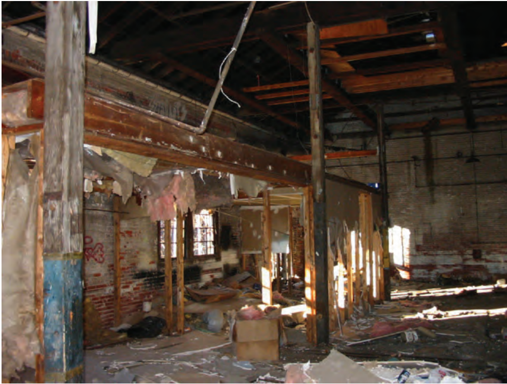
Interior of an existing structure within the Southern Opportunity Corridor.
