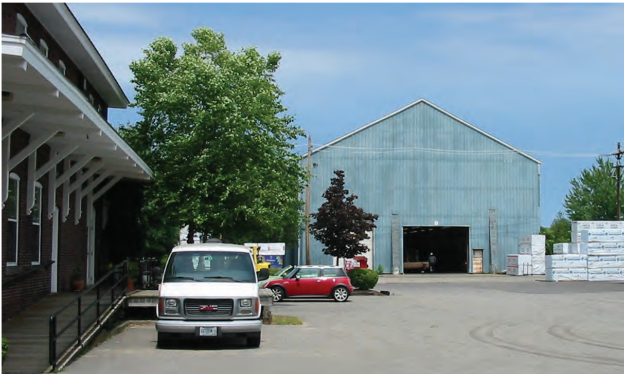
Looking north at the old train machine shops and assembly building.
