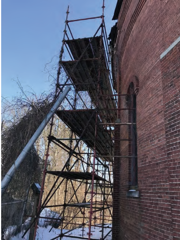
Photo #3-Exterior Shoring
