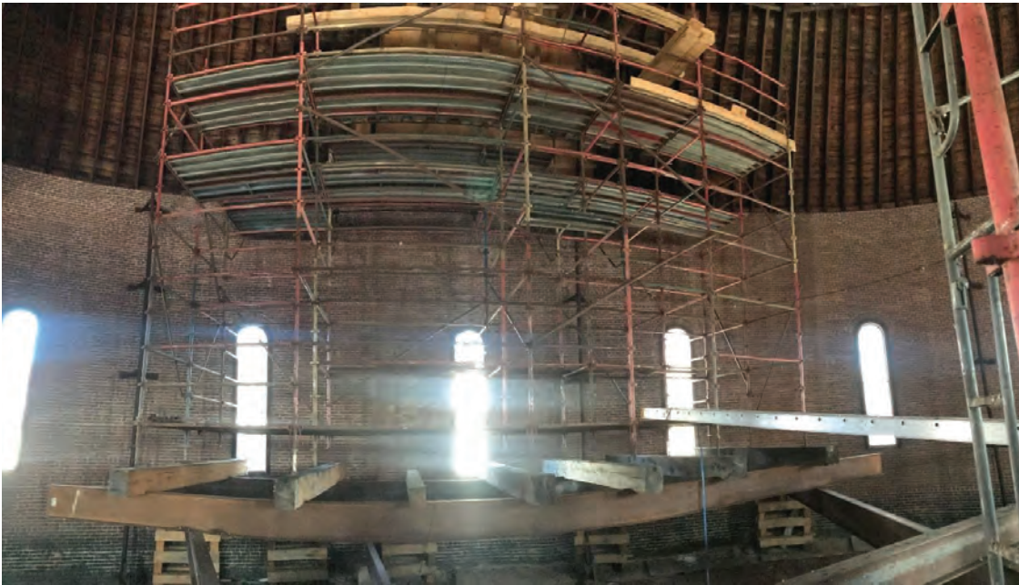
Photo #2-Shoring System at North Side
