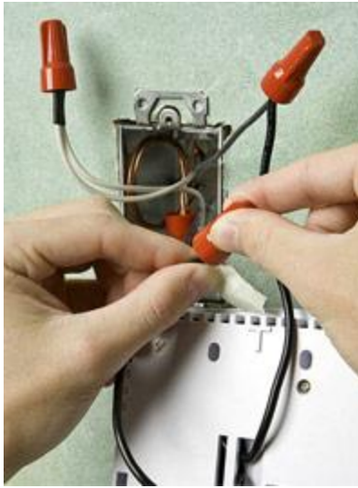
Figure 1. Line Voltage Residential Thermostat Wiring
