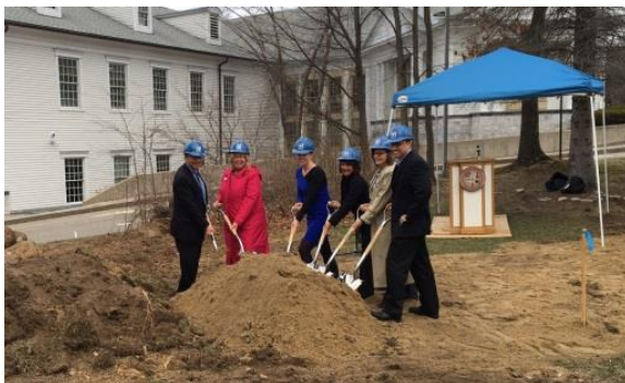
Bedford Library – Geothermal Groundbreaking
