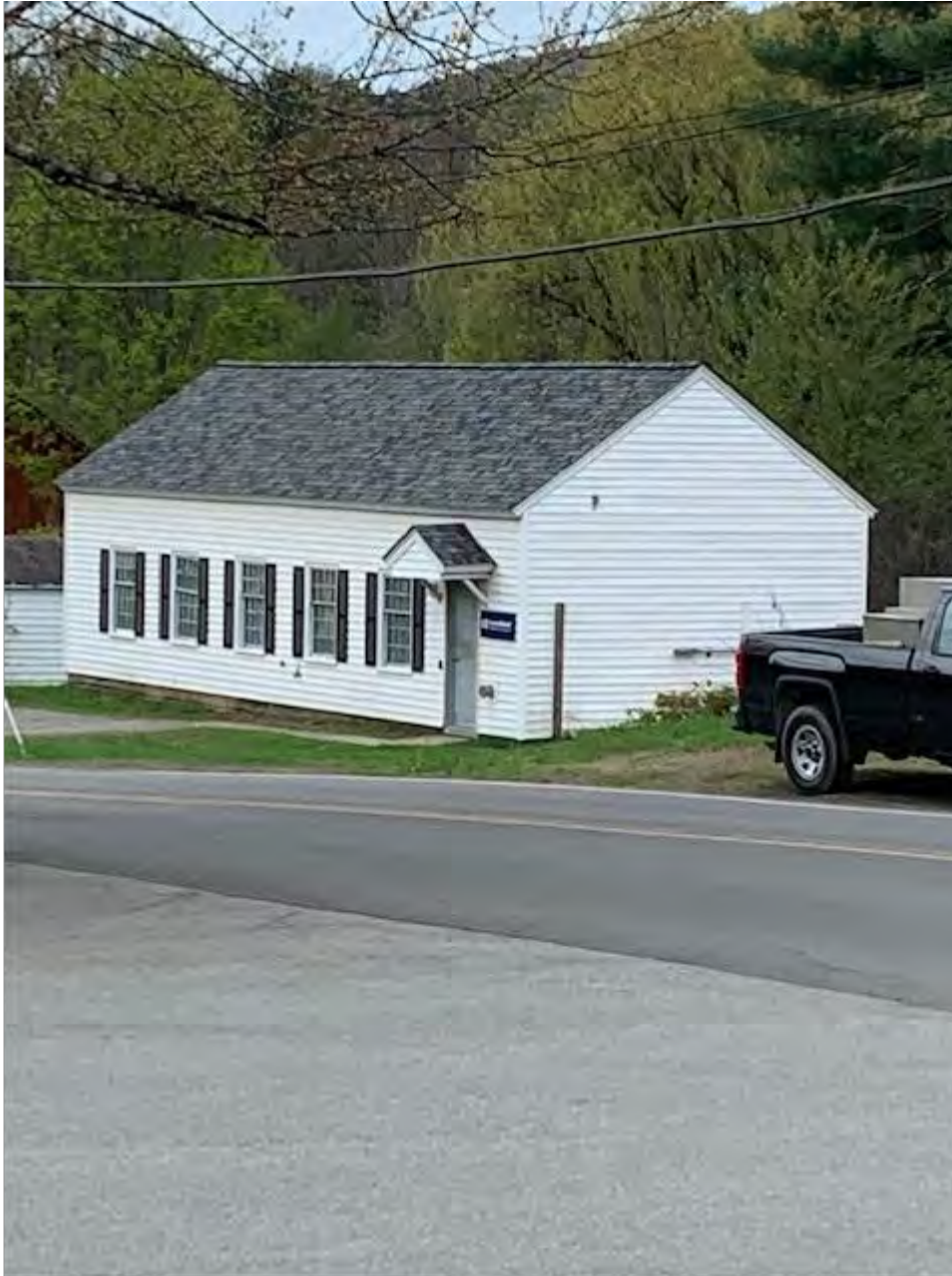
Consolidated Communications Building – near Village Store
